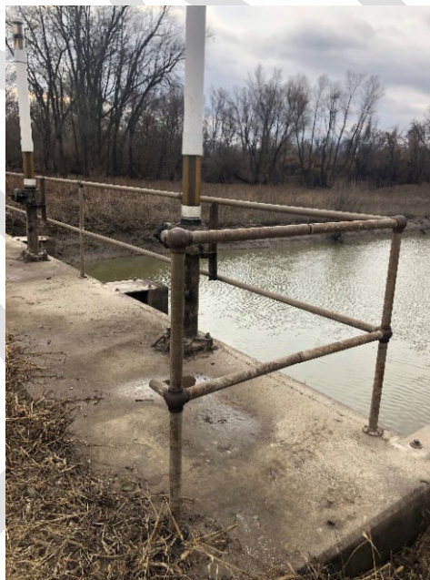
Photo 7. Typical guardrail on headwall structure
