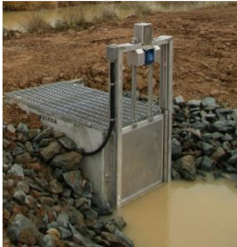
Photo 5. Automatic slide gate installed on box culvert opening
