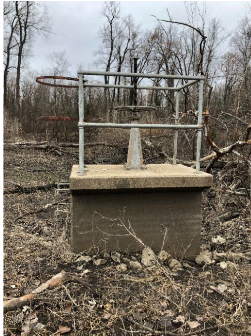
Photo 8. Typical guardrail and rungs on headwall structure
