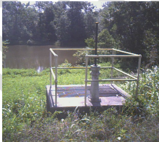
Photo 9. Example of metal grating on top of gatewell structure
