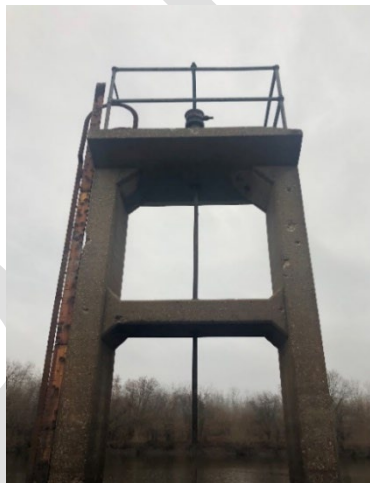
Photo 6. Slide gate installed on reinforced concrete headwall structure
